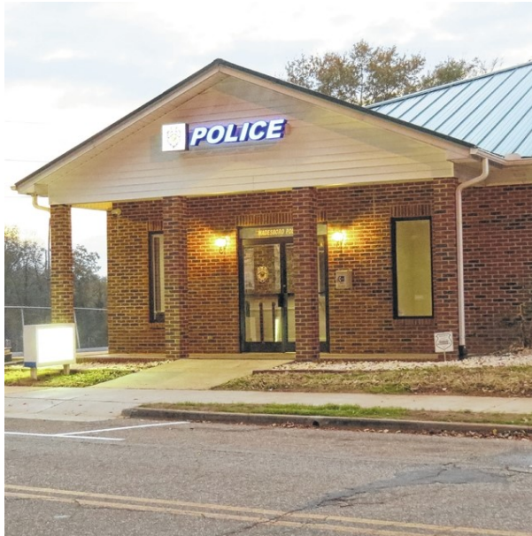
The Wadesboro Police Department's renovation project is an example of controlling the cost of government and doing more with less.
